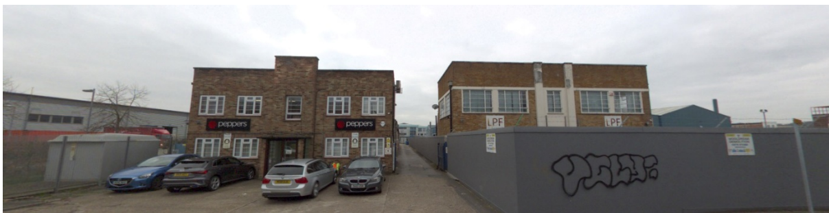
Context with adjacent building to right (access to Alfa Laval Car Park)
