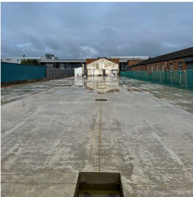
View to rear face of building from rear boundary
